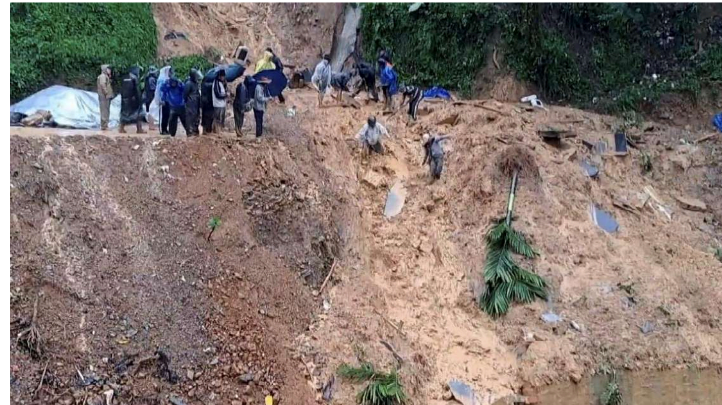
Debris being cleared after landslides due to incessant rains in the aftermath of Cyclone Remal, in Aizawl, Mizoram, May 30, 2024. File | Photo Credit: PTI
